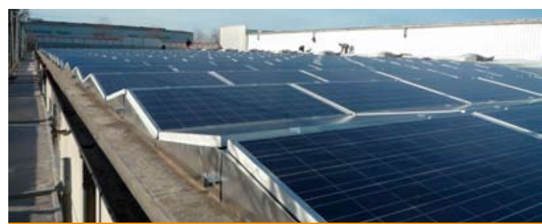
Roof view with side panels
